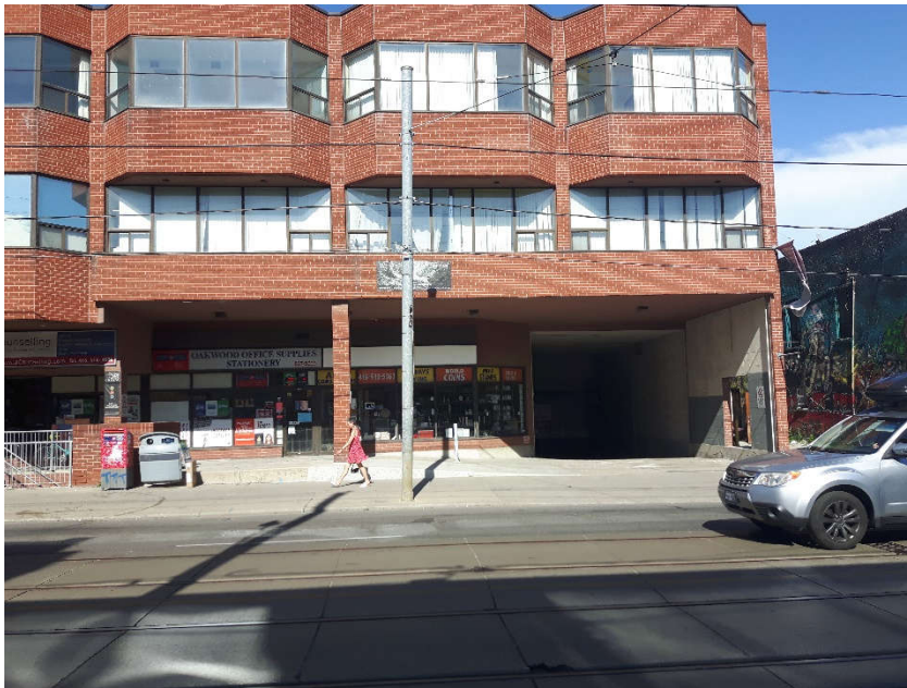
Image 2: View west to the apartment building at 2238 Dundas West.
