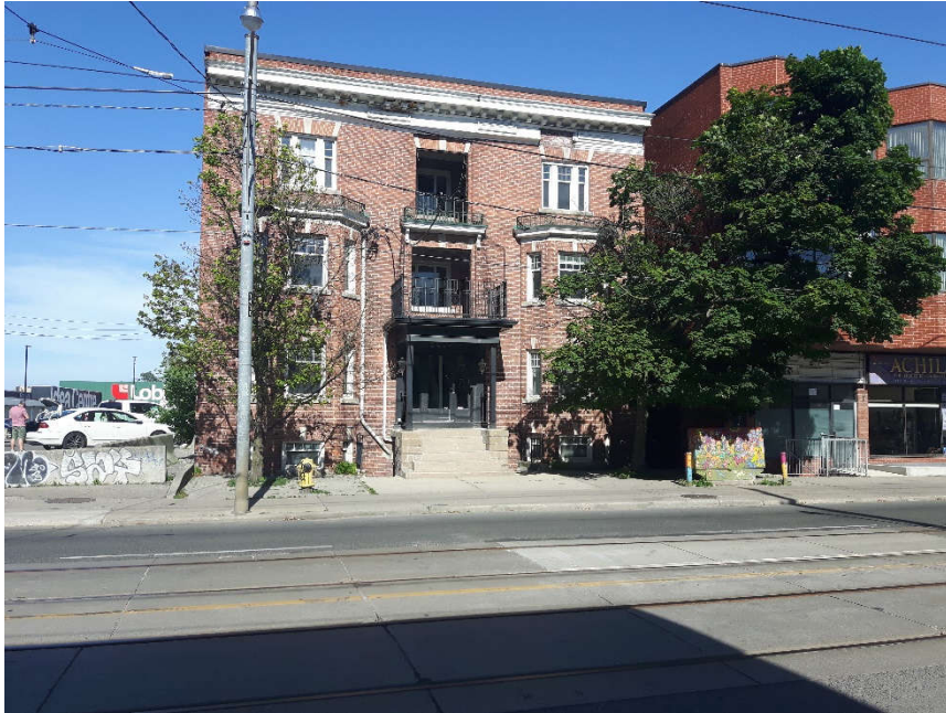
Image 4: View west to the apartment building at 2252 Dundas West.
